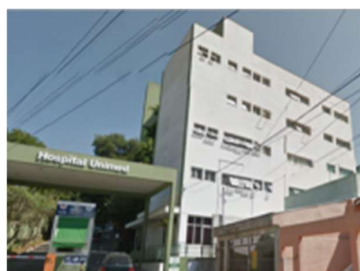
Hospital Unimed ABC
